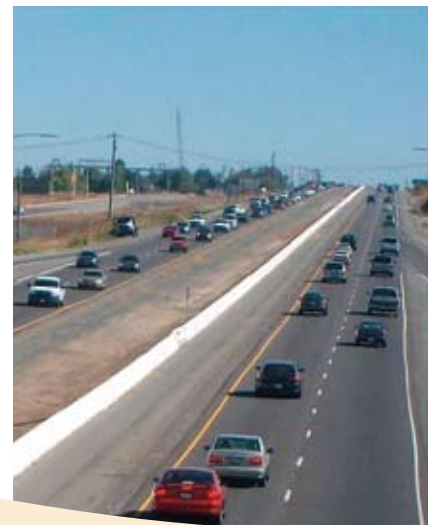
I-215 Widening Project in Murrieta
