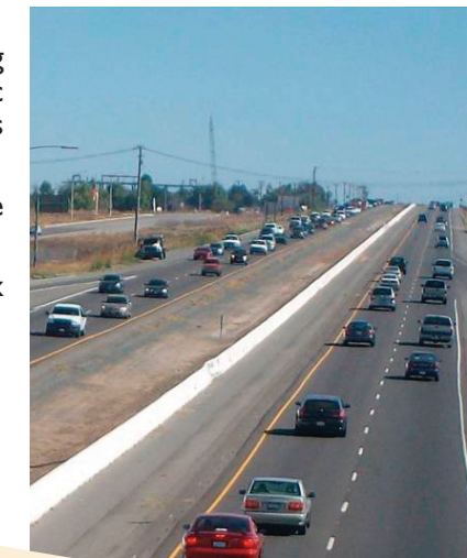
I-215 Widening Project in Murrieta
